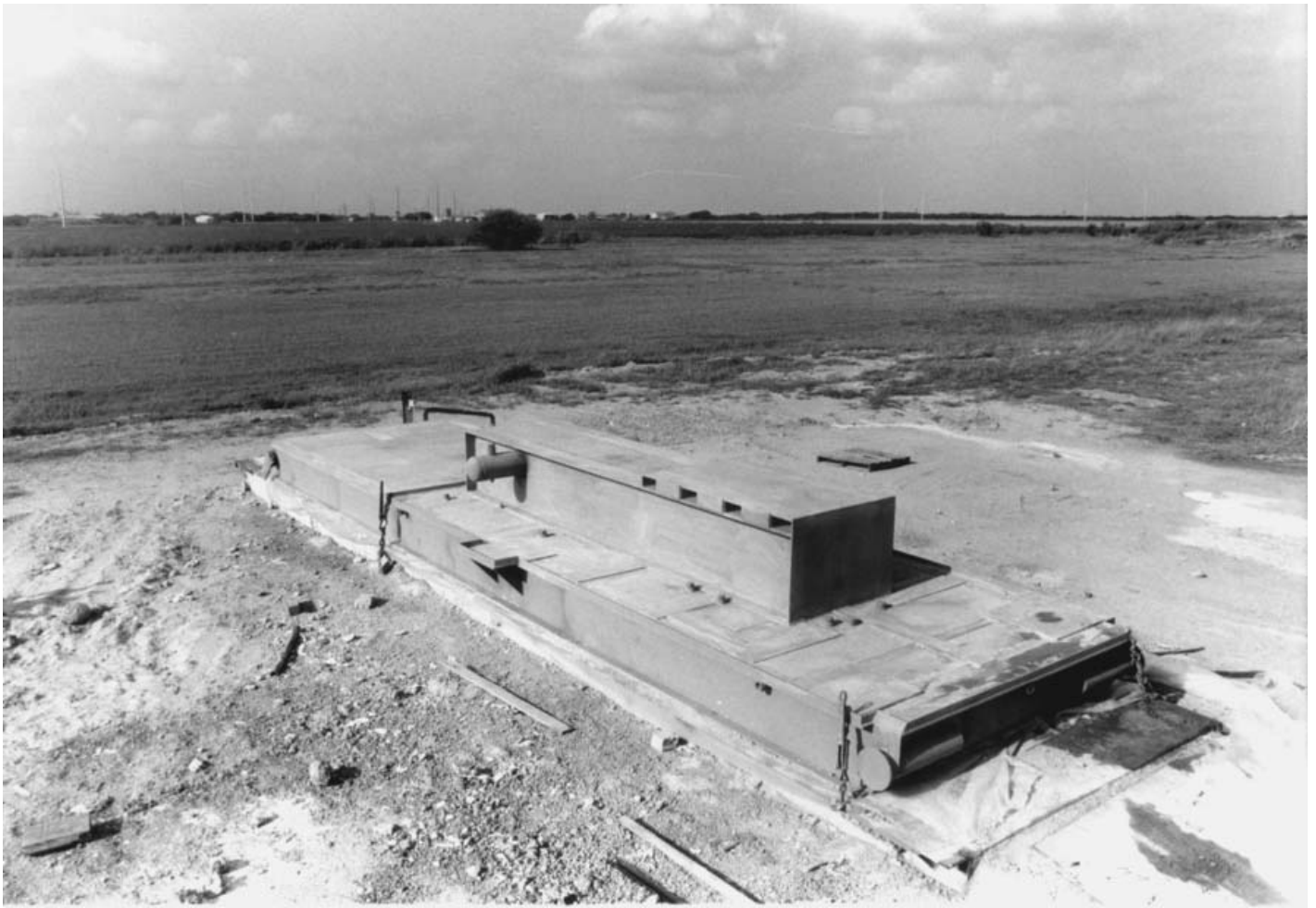
FIGURE 23.2 Typical skid design with concrete fill.
